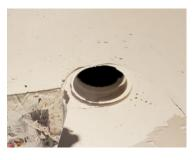
7. Apply as much joint compound as needed and begin to smooth out the surface.
