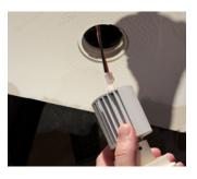
9. Connect wire from inside ceiling to back of the fixture.
