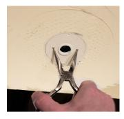
10. Insert fixture into screen socket. Insert the tip of a pair of pliers into the 2 notches and turn fixture COUNTER-clockwise to tighten fixture into place.
