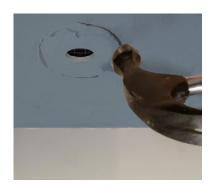
13. To remove fixture for servicing use a hammer to tap around the perimeter of where the hole is until the trim is free.
