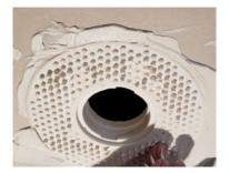
6. Align the screen hole with the hole in the ceiling and firmly press the screen into the wet joint compound. Make sure the joint compound comes out through the mesh holes and that the mesh is sitting flush against the ceiling.
