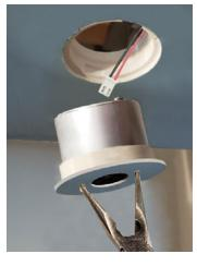
14. Using a pair of pliers, insert tips into notches then firmly turn the fixture CLOCKWISE to remove. Minimal damage to the painted plate makes re-installation a breeze.
