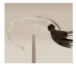
**13.** To remove fixture for servicing use a hammer to tap around the perimeter of the mesh screen to break apart the joint compound until the trim is free. The mesh screen can be reused of not severely damaged.
