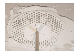
**10.** Firmly press the screen into the wet joint compound. Make sure the joint compound comes out through the mesh holes and that the mesh is sitting flush against the ceiling.
