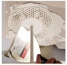
**11.** Apply joint compound over mesh screen. Allow to dry and reapply layers as necessary.
